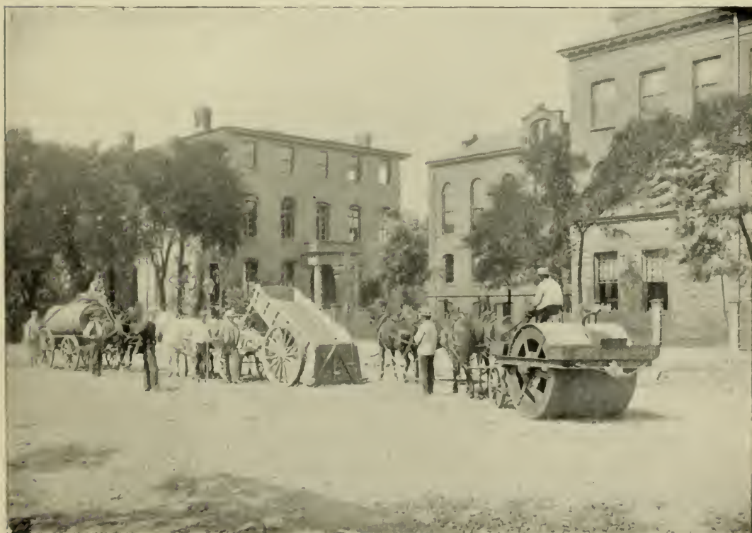
FIG. 2.—ROAD BUILDING BY U. S. DEPARTMENT OF AGRICULTURE FOR NEW JERSEY AGRICULTURAL COLLEGE AND EXPERIMENT STATION, NEW BRUNSWICK, N. J.
