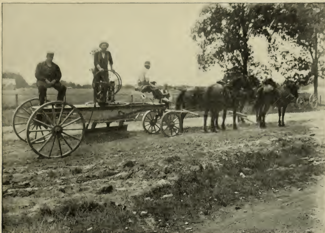
FIG. 1.—WORKING THE ROAD MACHINE.
